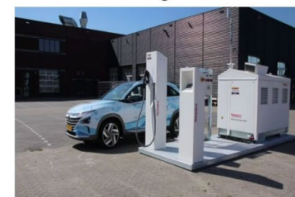
Containerised refuelling station
